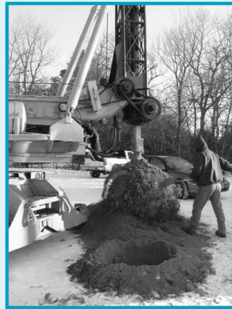
Construction begins at Nassahegan in late 2006
